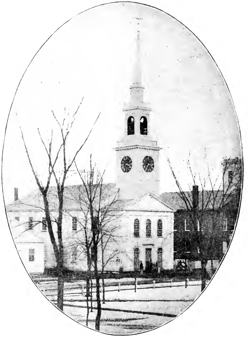
Third building of the town church, Westfield. Dedicated Jan. 1, 1806 It stood on the site of the present First Congregational Church
