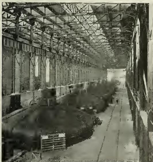
Fig. 5. Interior of Cedars Rapids Power House. Present equipment, nine 10,000 kv-a., 136-pole, 55.6 r.p.m., three-phase, 6600-volt generators. Ultimate equipment, eighteen similar units
