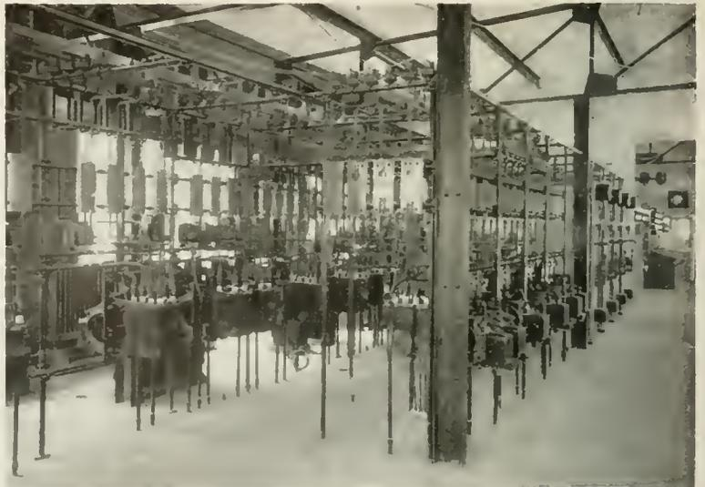
Fig. 15. View of 2300-volt Oil Switch and Bus Arrangement; also Series Lighting Panels
