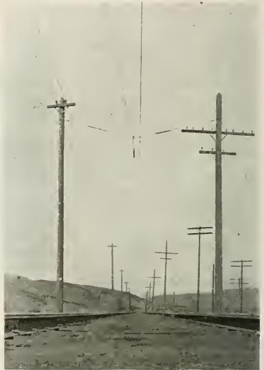
Fig. 10. The Arrangement of an Air Section Insulator
