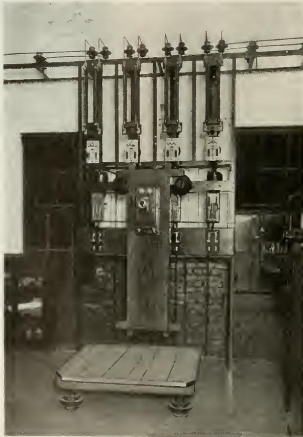
Fig. 7. Bank of Four High Voltage and Four Low Voltage Arresters at Boulevard Substation, Georgia Ry. & Pr. Co.
