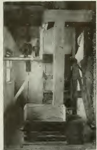
Fig. 4. 5-h.p., 60-cycle, 220-volt, Three phase, 1200-r.p.m. Motor Driving Flour Sifter
