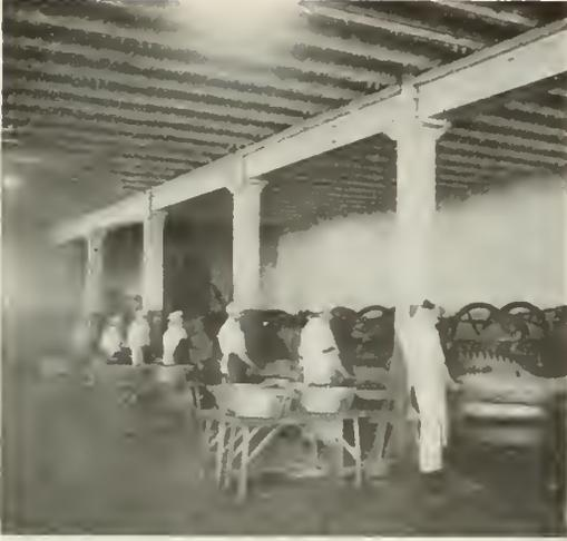
Fig. 45. 30-h.p., 900-r.p.m., Form K, 60-cycle, 220-volt Induction Motor Driving Battery of Sausage Chopping Machines
