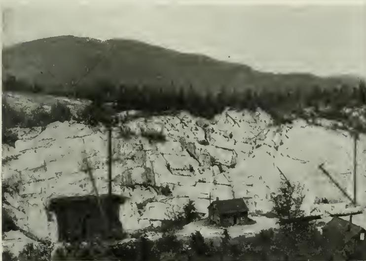
Fig. 5. Hollister Quarry—showing two typical quarry shafts and two motor-operated derricks
