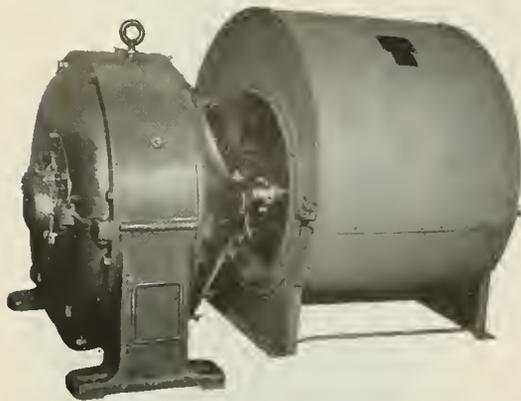
Fig. 17. MP-6-30-h.p., 620/775-r.p.m., 120-volt Motor
