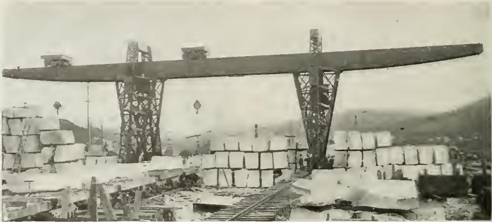
Fig. 7. Electrically-operated Gantry Crane serving block pile at West Rutland, Vt.
