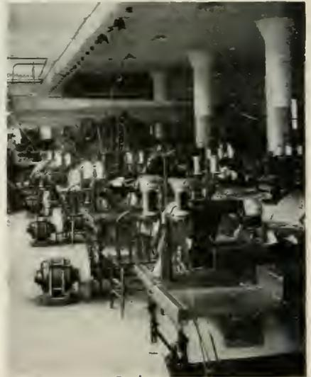
Fig. 22. 3-h.p., 1500-r.p.m., Motors Driving 20 Heavy Woolen Garment Sewing Machines
