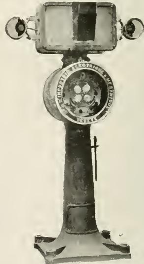
Fig. 8. A Column carrying a Switch, Voltmeter, and Ammeter as employed in the d-c. series system
