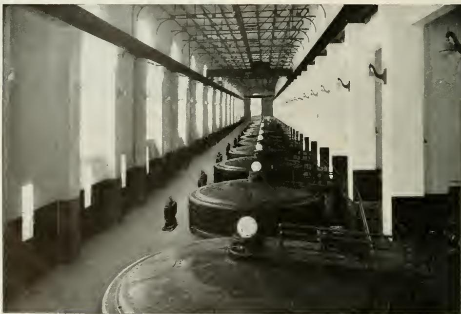
Fig. 3. 9000 Kv-a. Generators, Mississippi River Power Company, Keokuk, Iowa
