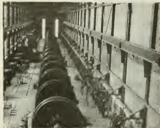
Fig. 6. Massena Substation of the Aluminum Company of America, containing eighteen 2500-kw. 360/500-volt Synchronous Converters. Power supplied from Cedars Rapids Manufacturing & Power Company
