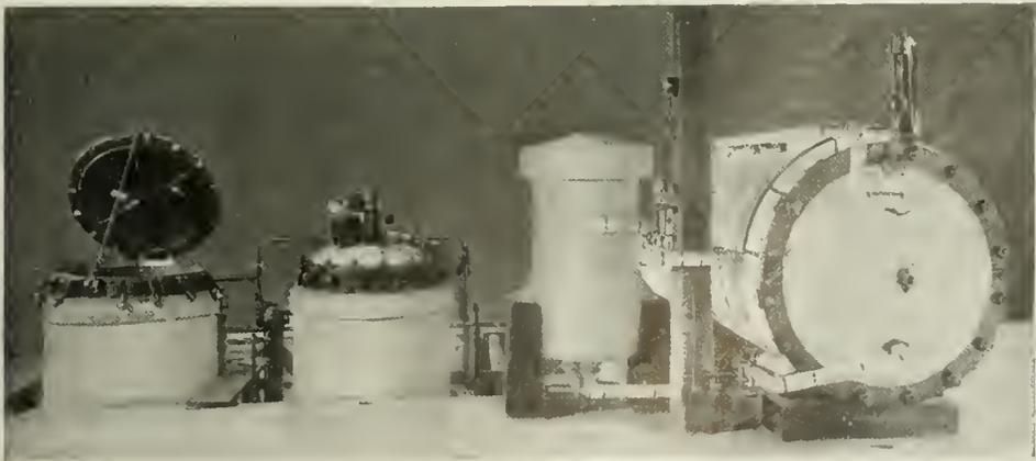
Fig. 6. A Three-foot by Four-foot Impregnating Set of Tanks at the Left and a Four-foot by Eight-foot Synthetic Resin Vulcanizer at the Right
