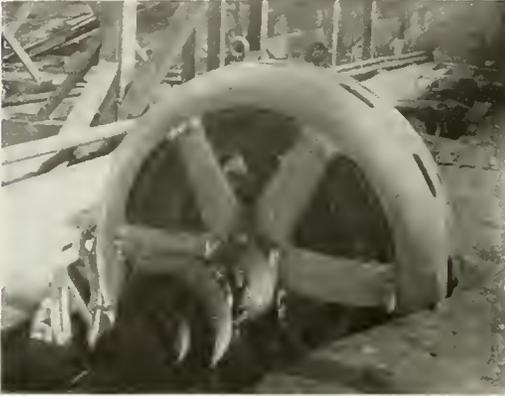
Fig. 11. 250-h.p., 240-r.p.m., Form M Induction Motor direct connected in line shaft—driving gang saws at Proctor Mill
