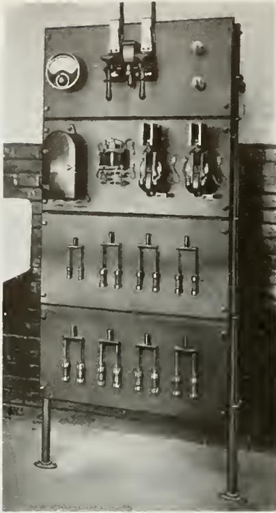
Fig. 10. Switchboard for Controlling the Heating of the Baking Oven
