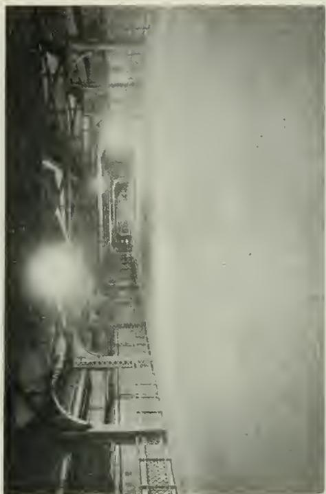
Fig. 7. Night View of Queensboro Bridge, New York City, lighted with 300-watt multiple type C Edison Mazda lamps in Novalux units with radial wave reflectors
