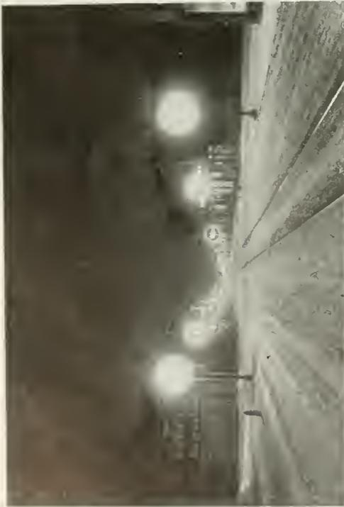
Fig. 10. Street in Corning, N. Y., showing illumination by 400 c.p. 15-amp. Edison Mazda C lamps with Novalux units
