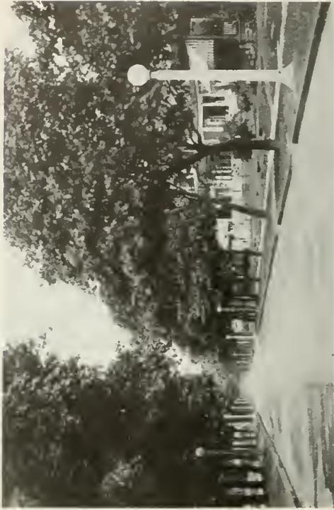
Fig. 11. Kenwood Avenue, Rochester, showing Mazda lighting with concrete lamp poles of the Rochester Railway & Light Company
