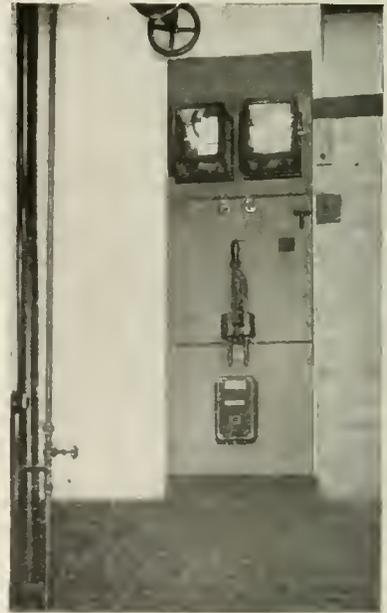
Fig. 2. Control Board, Showing Operating Lever of the Oil Switch and the Curve-drawing Instruments
