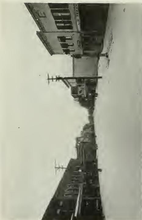
Fig. 8. Dansville, N. Y., 600-c.p., 20-amp. Edison Mazda type C lamp with Novalux units
