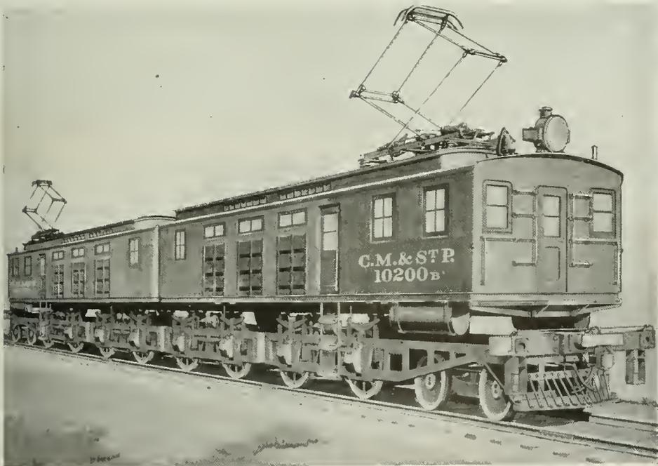
Fig. 13. Chicago, Milwaukee & St. Paul Electric Locomotive, 21 of which are now under construction.
