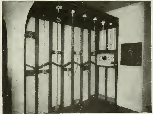
Fig. 5. Section of Wall and Roof of House showing how Wiring and Wiring Devices are Installed, Exhibit of General Electric Company, Palace of Manufactures
