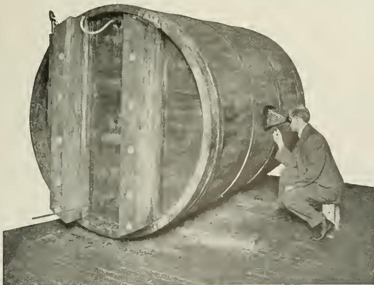
Fig. 1. Cask for Study of Variation of Spark-Over and Corona Voltage with Air Density or Altitude
