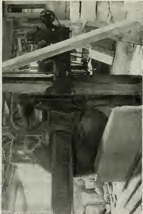
Fig. 14. Diamond Saw driven by a 25-h.p. motor with 3-h.p. motor on feed
