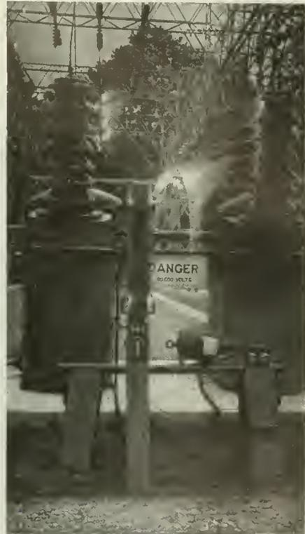
Fig. 6. Telephone Arrester Operating on 118,000 Volts from Power Line
