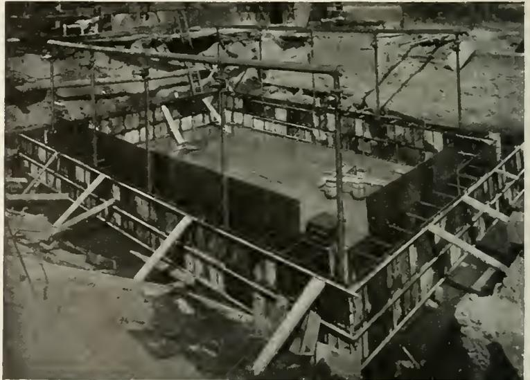
Fig. 1. Lower Forms for Impregnating Pit Walls set in place
