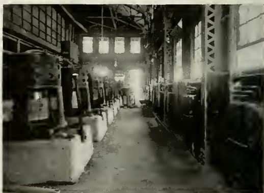
Fig. 12. 75-h.p., 500-r.p.m., Form K, 25-cycle, 550-volt Induction Motor Belted to Fuller Mills in Crusher House for Cement
