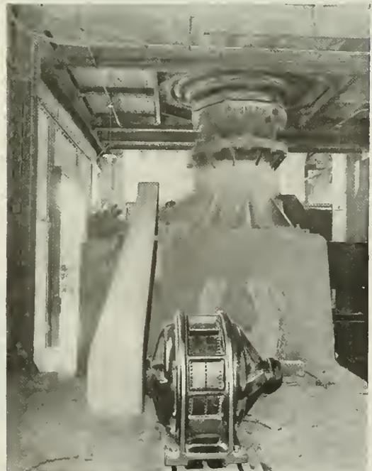
Fig. 62. 50-h.p., 900-r.p.m., Form K, 440-volt Induction Motor Driving Crusher
