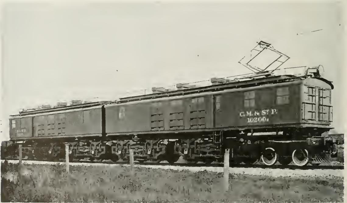
Fig. 2. The First 3000-volt, 282-ton, C., M. & St. P. Locomotive on the Eric Test Tracks of the General Electric Company
