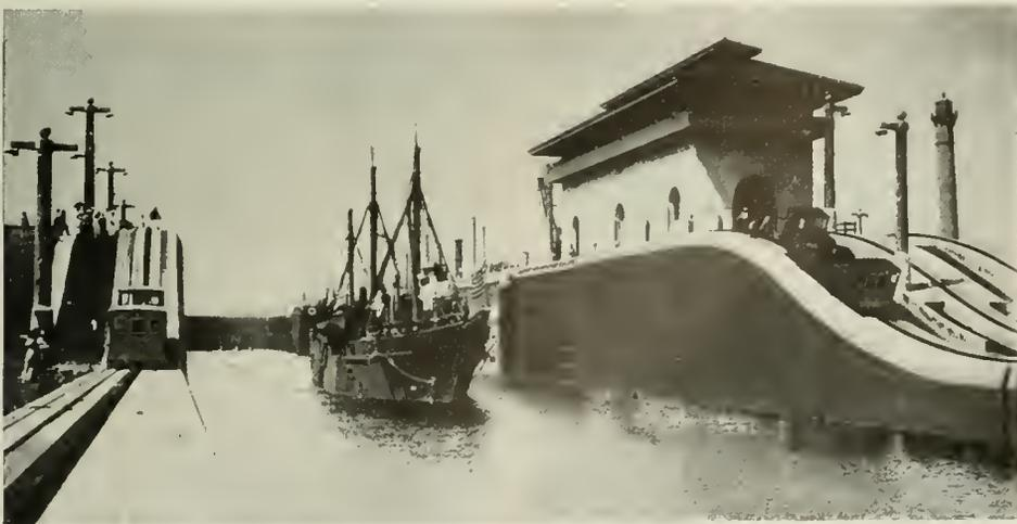
Fig. 13. The "Severn" Leaving the Upper East Chamber in the Tow of Electric Locomotives
