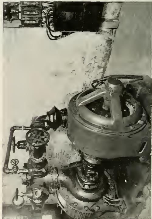
Fig. 17. 100-h.p., 1800-r.p.m., Form K Motor Direct Connected to Centrifugal Fire Pump in Fertilizer Plant
