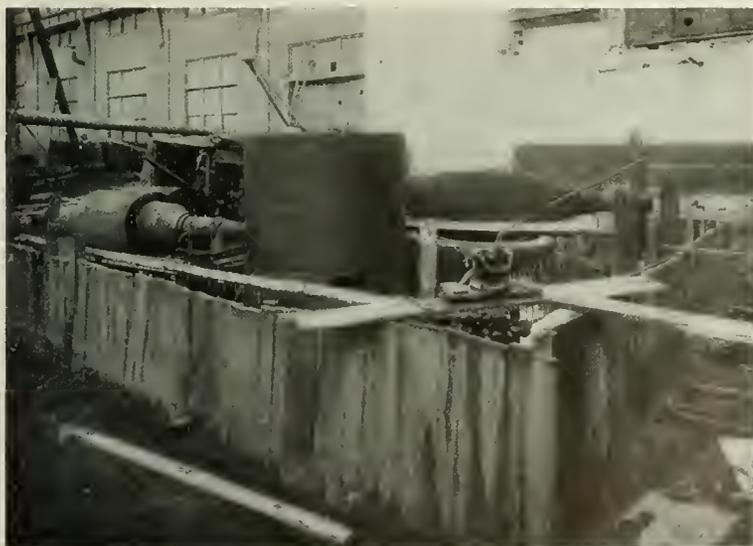
Fig. 2. Loads as placed on the Tank to Facilitate Sinking it into place
