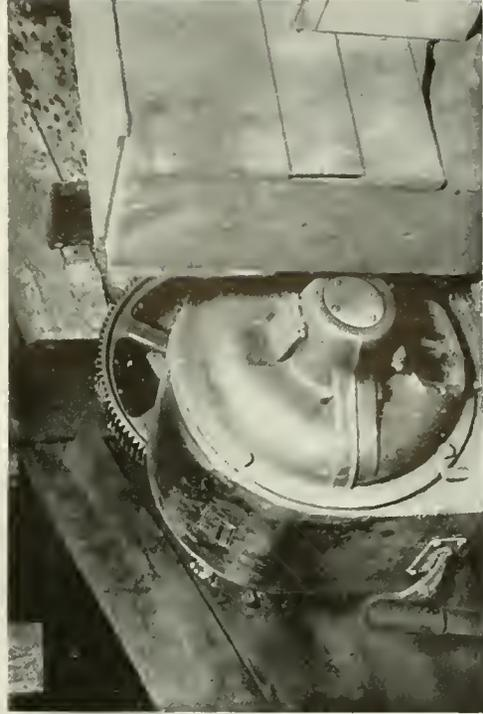
Fig. 38. 25-h.p., 900-r.p.m., 440-volt, 60-cycle, Three-phase, Form K Mining Type Induction Motor Installed on Coal Crusher
