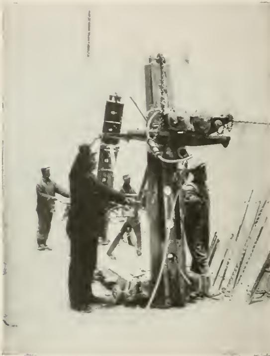
Fig. 4. Drill Mounted on Gadder Post Operating in a Marble Quarry
