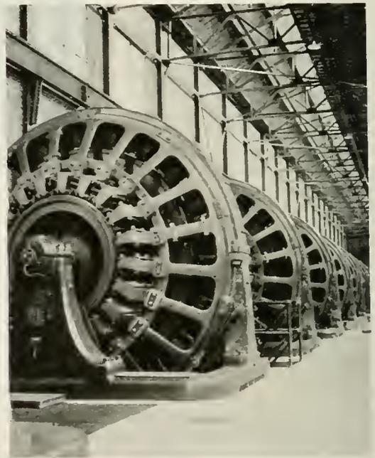
Fig. 4. The Direct-Current Ends of the Converters as installed, showing the moulded asbestos pieces on the brush-holders
