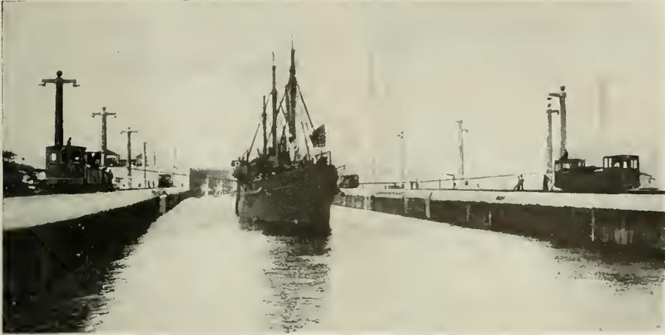
Fig. 12. Four Towing Locomotives Attached to the Submarine Tender "Severn" in a Gatun Lock Ready for Lowering the Water-Level. A group of submarines may be seen at the far end of the lock
