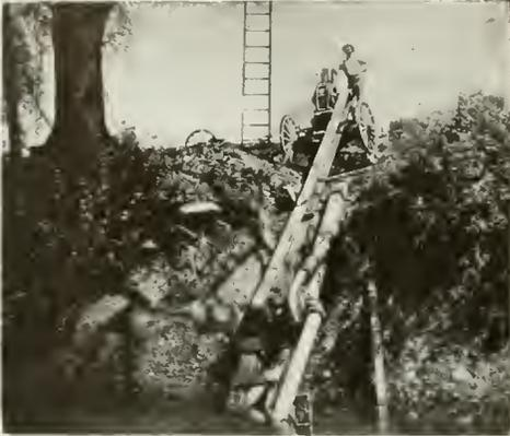
Fig. 9. Portable Motor and Six-Inch Centrifugal Pump for Irrigating Forty Acres of Alfalfa in California
