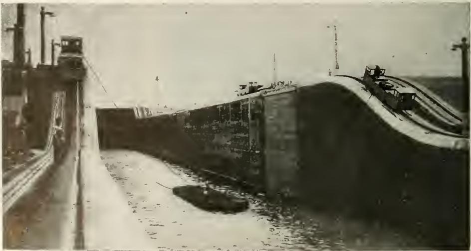
Fig. 11. The First Trail Tow with the Barge at the Second Level of the Gatun Locks, Rear Locomotives Ascending the Incline. The water in this middle lock (second level) is shown at sea level, a condition not obtained in regular operation. This trial was made to demonstrate that the tow lines would clear the lock walls
