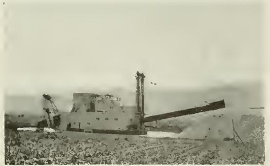
Fig. 4. Electrically-operated Gold Dredge
