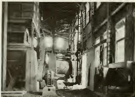
Fig. 11. 50-h.p., 500-r.p.m., Form K, 25-cycle, 550-volt Motor Driving Ball Mills in Plant
