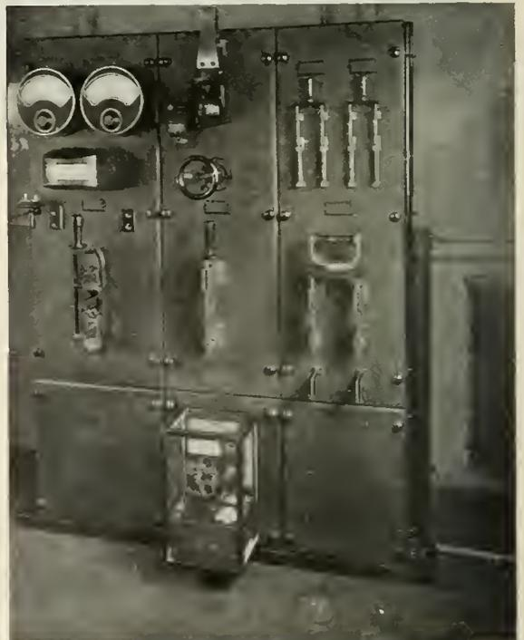
Fig. 3. The Control, Feeder and Starting Panels (left to right) of the Portable Substation Switchboard
