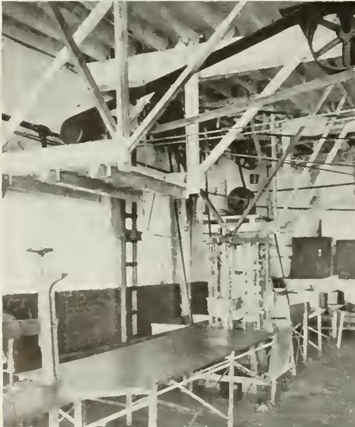
Fig. 47. 25-h.p., 1000-r.p.m. and 10-h.p., 750-r.p.m., 220-volt Motors Driving Vacuum Pump, Meat Chopper, Hasher and Corn Beef Filler
