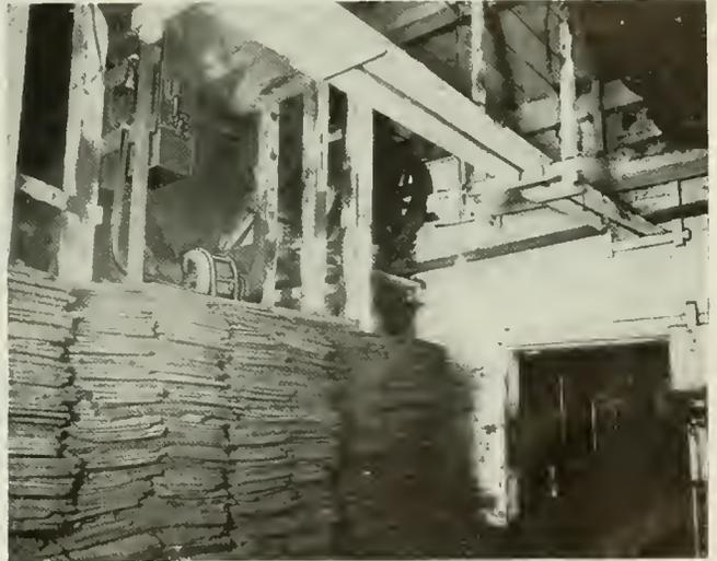
Fig. 14. 35-h.p., 1800-r.p.m. Motor Driving Cake Mills in Cotton Seed Oil Plant
