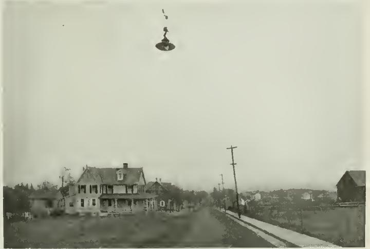
Fig. 2. Day View of Washington Street, Sellersville, Pa., showing G-E eye suspension fixtures equipped with concentric reflectors, prismatic refractors and 100-c.p. 6.6-amp. series Mazda lamps
