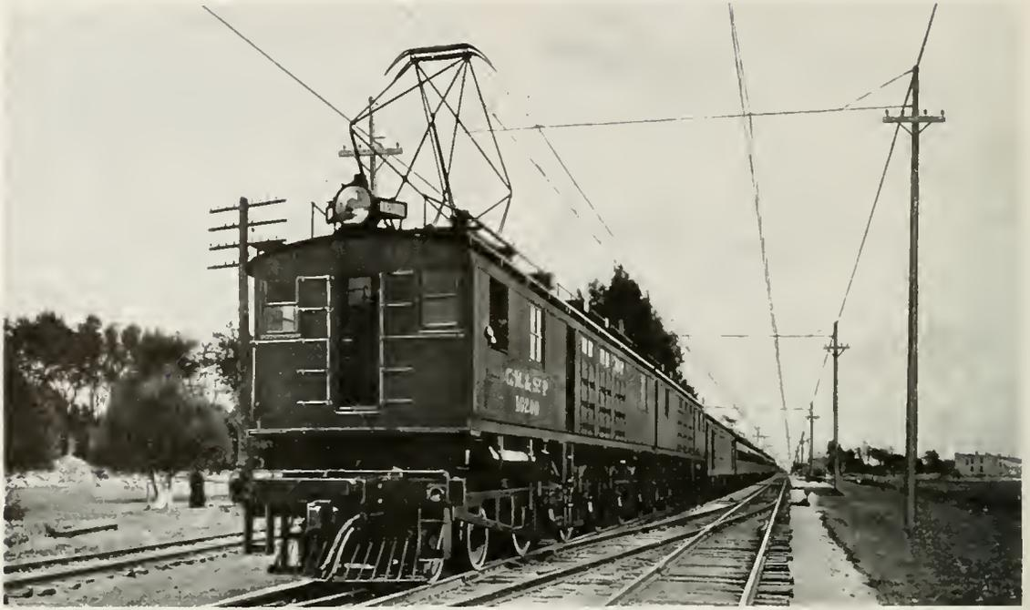
Fig. 1. The First 3000-volt, C., M. & St. P. Locomotive shown Coupled to the "Olympian," the famous transcontinental train between Chicago and Tacoma
