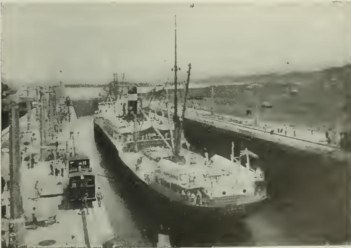
Fig. 9. The "Ancon" Entering the Upper Gatun Lock from the Middle West Chamber under the Tow of Electric Locomotives
