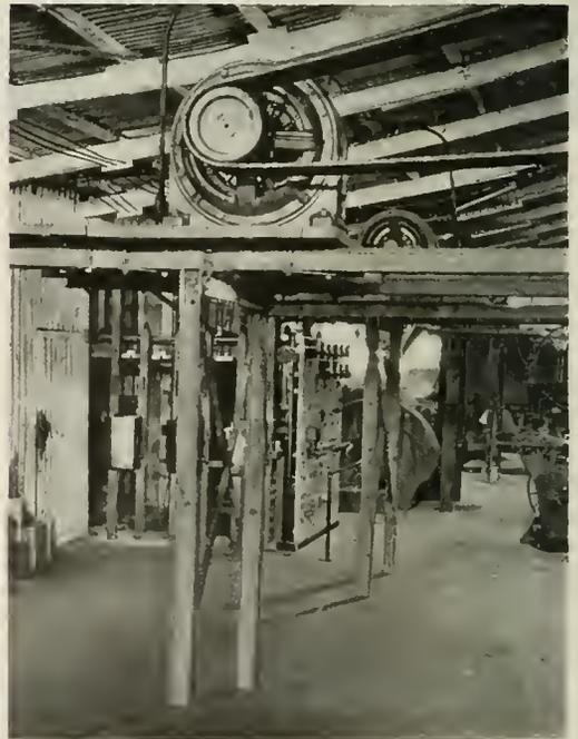
Fig. 6. Method Employed in Mounting the Motors
