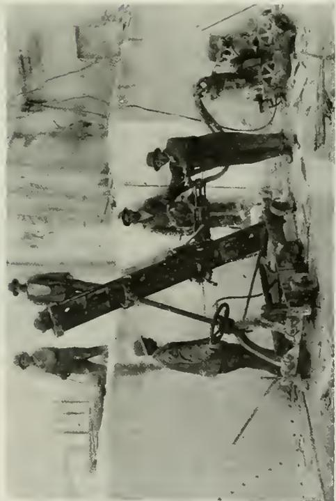
Fig. 3. Electric-Air Drill driven by a  $5\frac{1}{2}$ -h.p., 1800/900-r.p.m., 220-volt Form KT induction motor
