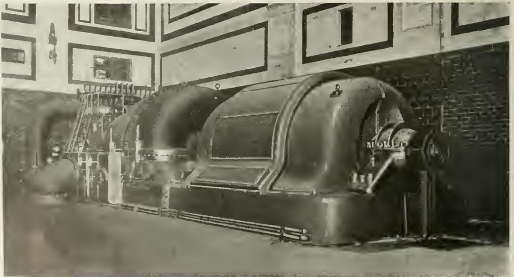
Fig. 1. 30,000-Kw. Steam Turbo-Generator, New York Edison Co.
