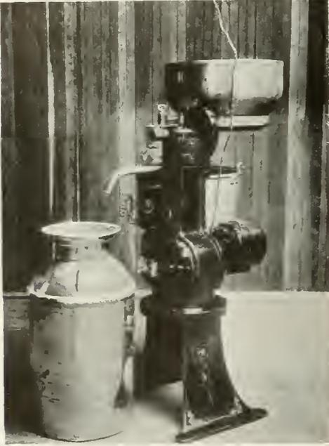
Fig. 14. Cream Separator Driven by  $\frac{1}{2}$ -h.p. Motor
