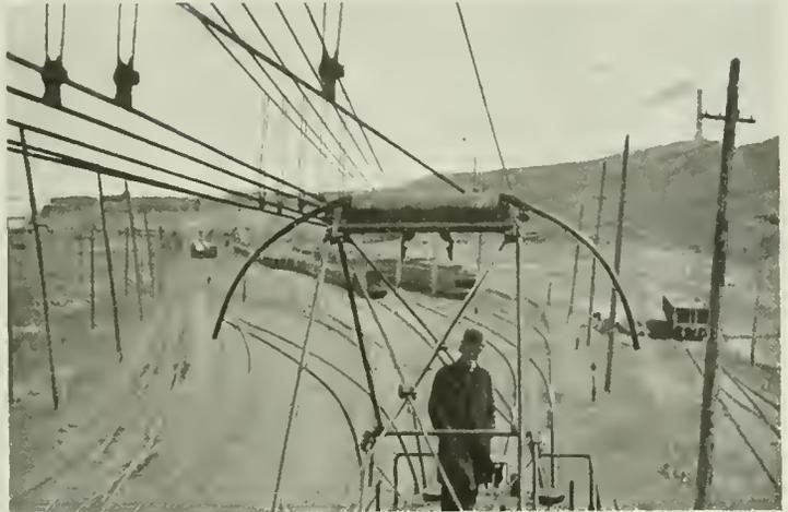
Fig. 8. Pantograph in Contact with Six Trolley Wires at a Switching Point
