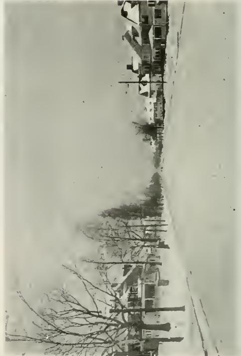
Fig. 12. Lake Avenue, Rochester, N. Y., showing ornamental post units built by Rochester Railway & Light Company, 1000-c.p., 20-amp. Edison Mazda C lamps
