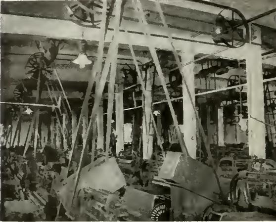
Fig. 19. Weave Room Operated by Mechanical Drive
